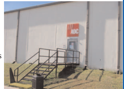
Entrance to the ADC facility in Lexington, SC.
